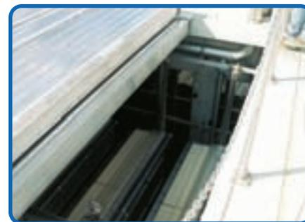
multifunctional permeate pumps as opposed to separate permeate and back-pulse pump systems. Flux maintenance is achieved in the hollow-fiber system by relaxing, air pulsing, regular back-pulsing or chemical back-pulsing, regular chemical maintenance cleaning and periodic recovery cleaning. The surrounding systems include onsite chemical pump systems, chemical storage, back-pulse pumps, back-pulse tanks and tank-drain pumping capabilities for higher strength chemical recovery cleaning.
